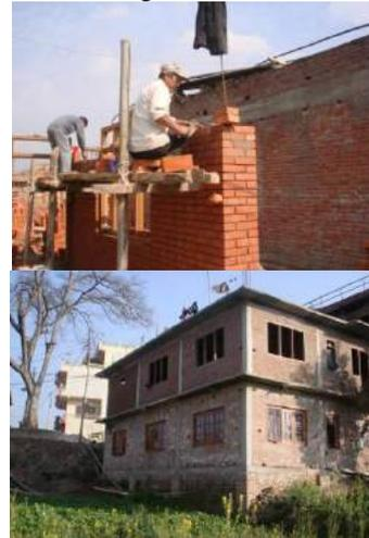
Figure 6. Typical Non-Engineered Buildings in Nepal
