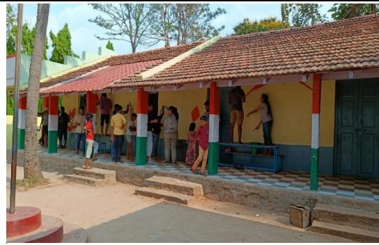
PAINTING THE WALLS
